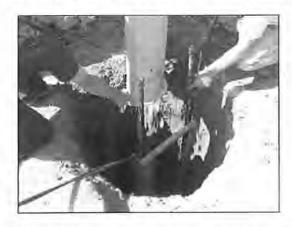
Fine aggregate in concrete is being replaced by bottom ash in a demonstration project at the new Medical Office Building in Marion, Illinois.
