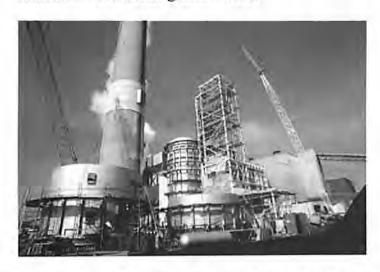
Wet scrubbers on CWLP's Dallman Power Station trap sulfur dioxide in the flue and chemically change it to environmentally-friendly gypsum.
