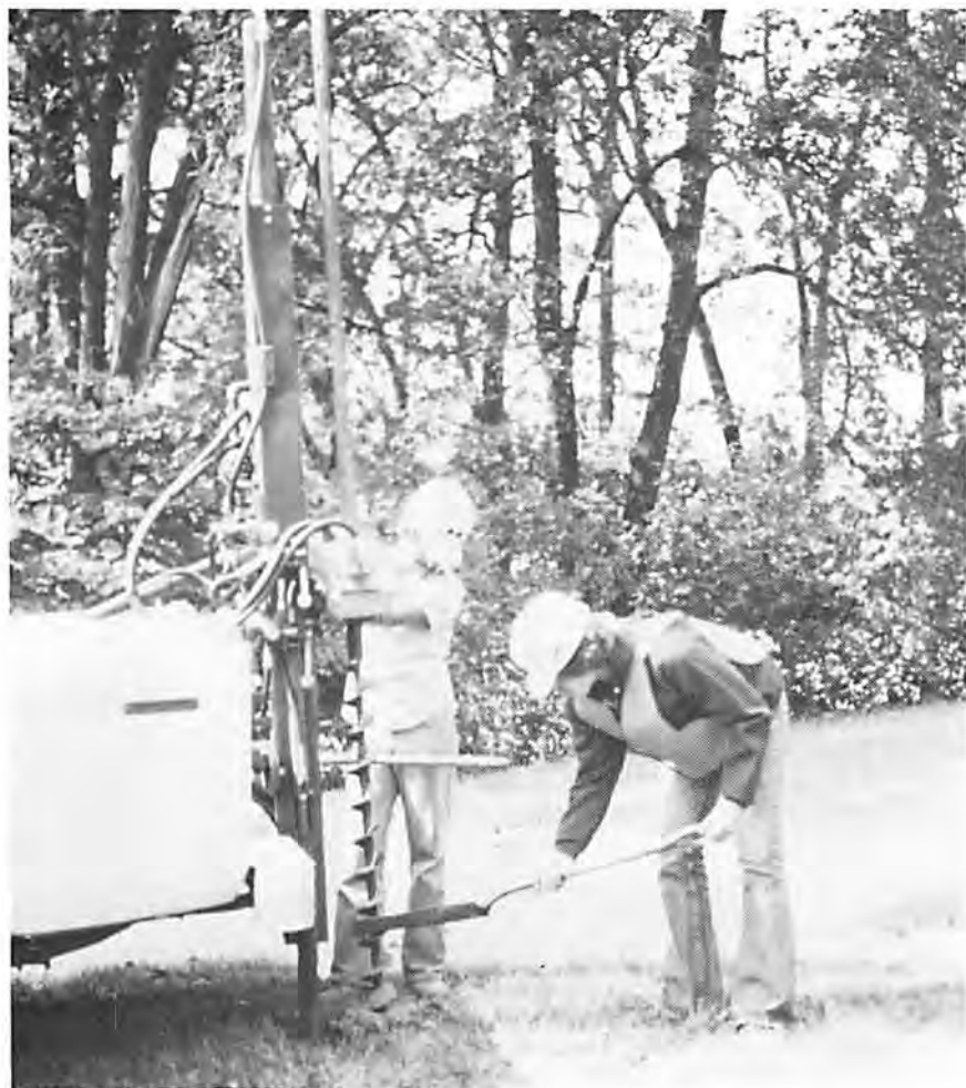
Fig. 5 — Peabody's Surface Drill with Auger and Kelly Bars.
