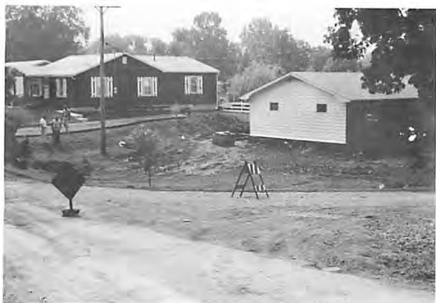
Fig. 1 — Two homes in the Williamson County village of Energy where mine subsidence effects were abated by supporting the buildings independent of the ground.
