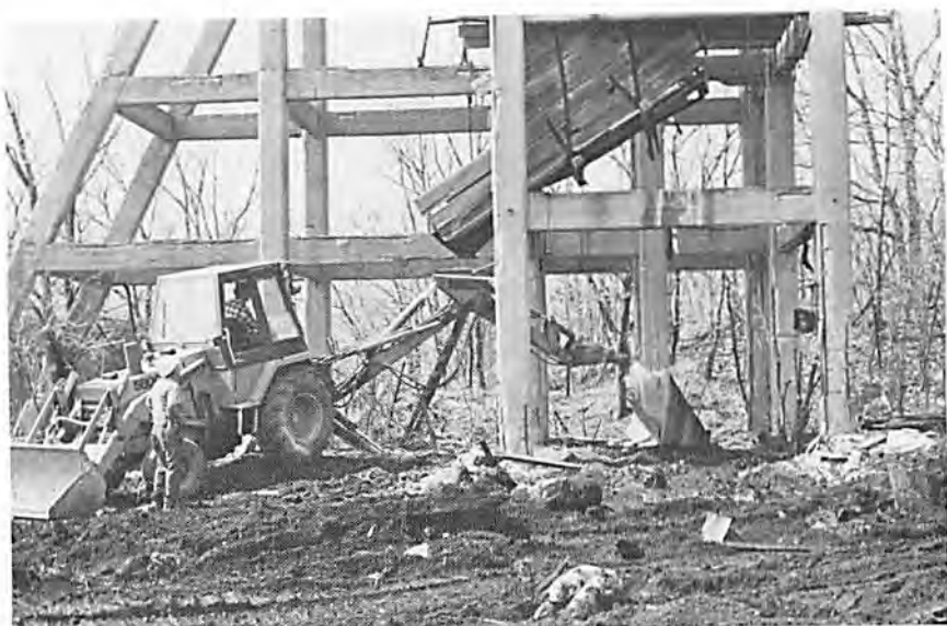
Fig. 2 — In Carlinville, the concrete tibble of the Old South Mine was demolished prior to filling two mine shafts and reclaiming the site.
