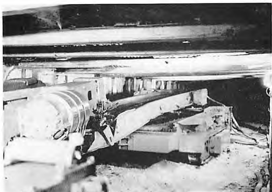
A 16-ft. bridge conveyor serves to tie the continuous miner to the extensible conveyor
