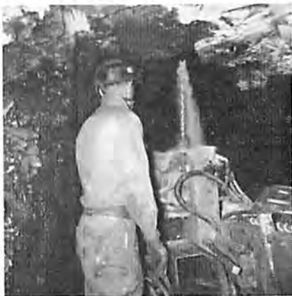
The bolting pattern is staggered down the room on four-ft. centers and 2¼ ft. from the rib, considering only lateral dimension. Approximately one bolt per ft. in a 17½-ft. wide room is used
