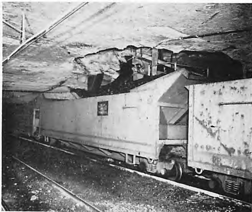
Large capacity mine cars in use today require scheduled maintenance, such as proper lubrication and frequent inspections.
