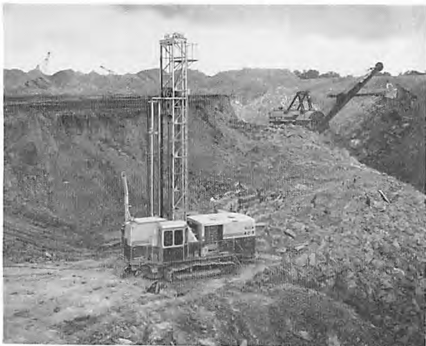
The 40-R above drills 6¾- to 9-in. holes; the larger 50-R, 9¾- to 12¼-in. holes.
