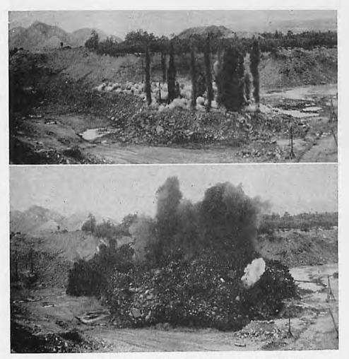
Fig. 3. Sequence views of a typical blast initiated from the top of a vertical hole
