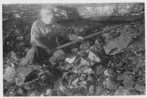
Fig. 5. Face fall shows the excellent breakage by Chemechol
