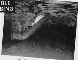
MineVent Tubing on blower fan at Orient Mine No. 3
