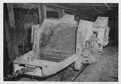
Track mounted shuttle car hauls material to top of glory hole
