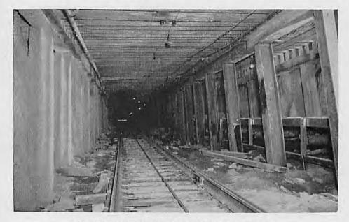
View during construction showing track and belt compartments
