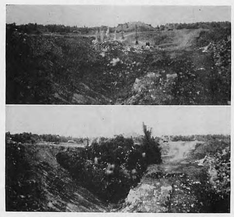
Fig. 4. An anthracite blast detonated with milli-second delays at the bottom of the holes
