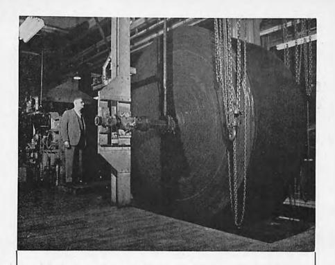
Yes! It's a "Rotocured" conveyor belt continuously uniform throughout its entire length. Only possible through BWH Exclusive "Rotocure" Process of Continuous Vulcanization.
