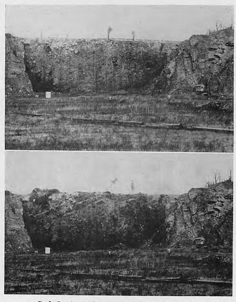
Fig. 2. Two views at 1/3 second intervals show progress of detonation
