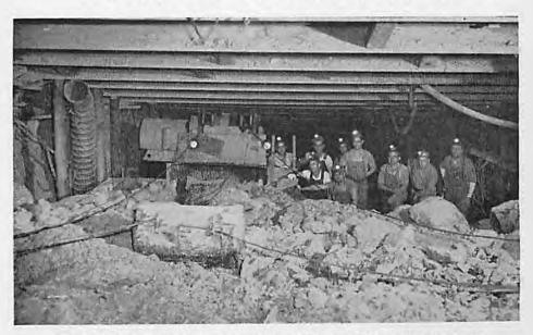
Slusher bucket drags rock into loading machine which in turn discharges into shuttle car
