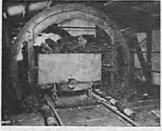
ROTARY DUMPS for use in mines where large lumps make the use of drop bottom, side, or end dump cars prohibitive.
