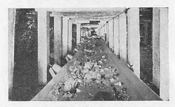
Coal being carried by Manhattan Homocord Conveyor Belt on gathering line in underground mine.
