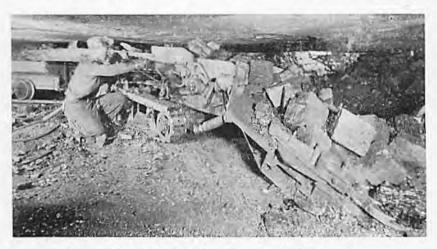
Low coal is mined efficiently with tractor loading machine.
