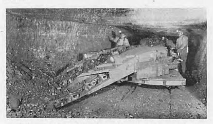
Track mounted mechanical loader working under ideal seam conditions.
