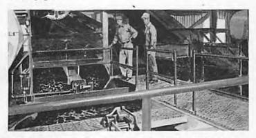
Washer section . . . coal preparation plant where two McNally-Nortons wash coal 6 x 0. Larger sizes, unwashed, are loaded direct after hand picking or are crushed, washed, and reclassified for loading.
