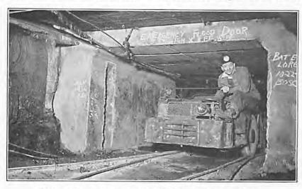
Figure 12.—Saxton emergency flood door, haulage-road side.
