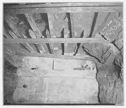
FIGURE 9.—Typical timbering at Saxton primary bulkhead.
