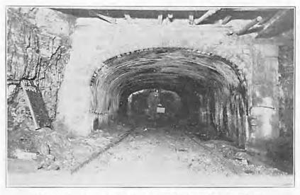
Figure 10,—Concrete arch in front of Saxton primary bulkhead.
