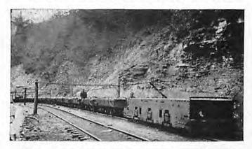
20-Ton, Three Motor, Haulage Locomotive with Loads.
