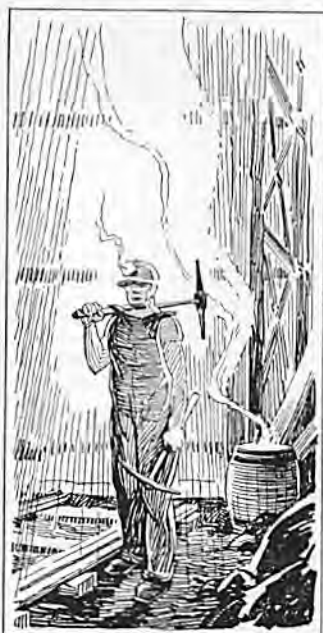
Ventilation was obtained by keeping a powder keg full of coals burning at the foot of the upcast.
