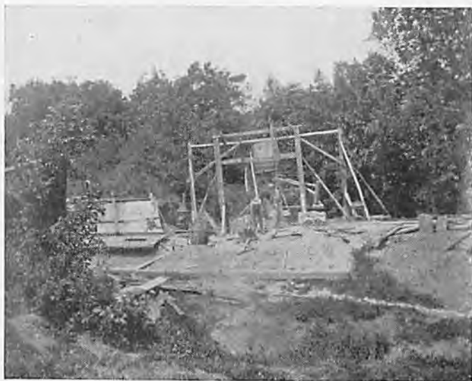
Brophy's mine, Shelby County, Illinois. A gin hoist and blind horse for the motive power. In the foreground, left, is the loading platform. Note the loaded mine car to the right of the shaft. The gin sweep with the horse in the shafts can be seen back of the car. The drum is above the men.
