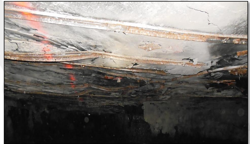
Underground Roof Condition w/InStaL Bolts & “TT” Anti-Friction Washer
