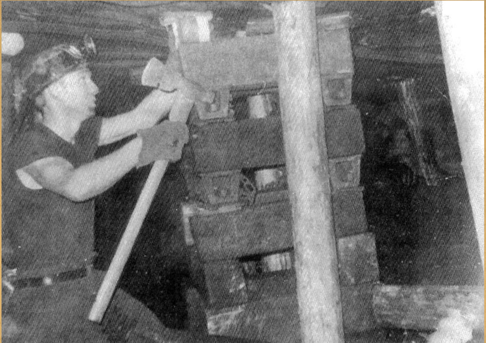
Building Wooden Chocks on the Longwall
